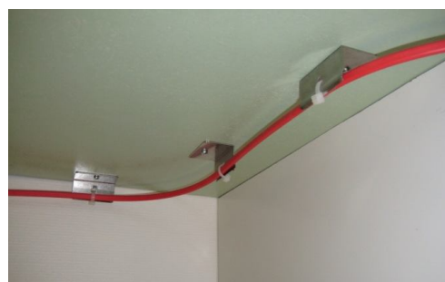
Sensor cable installed with brackets and straps
